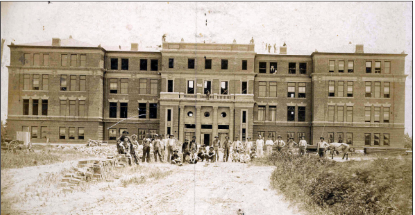
Pittsburg State University Russ Hall under construction, 1907
